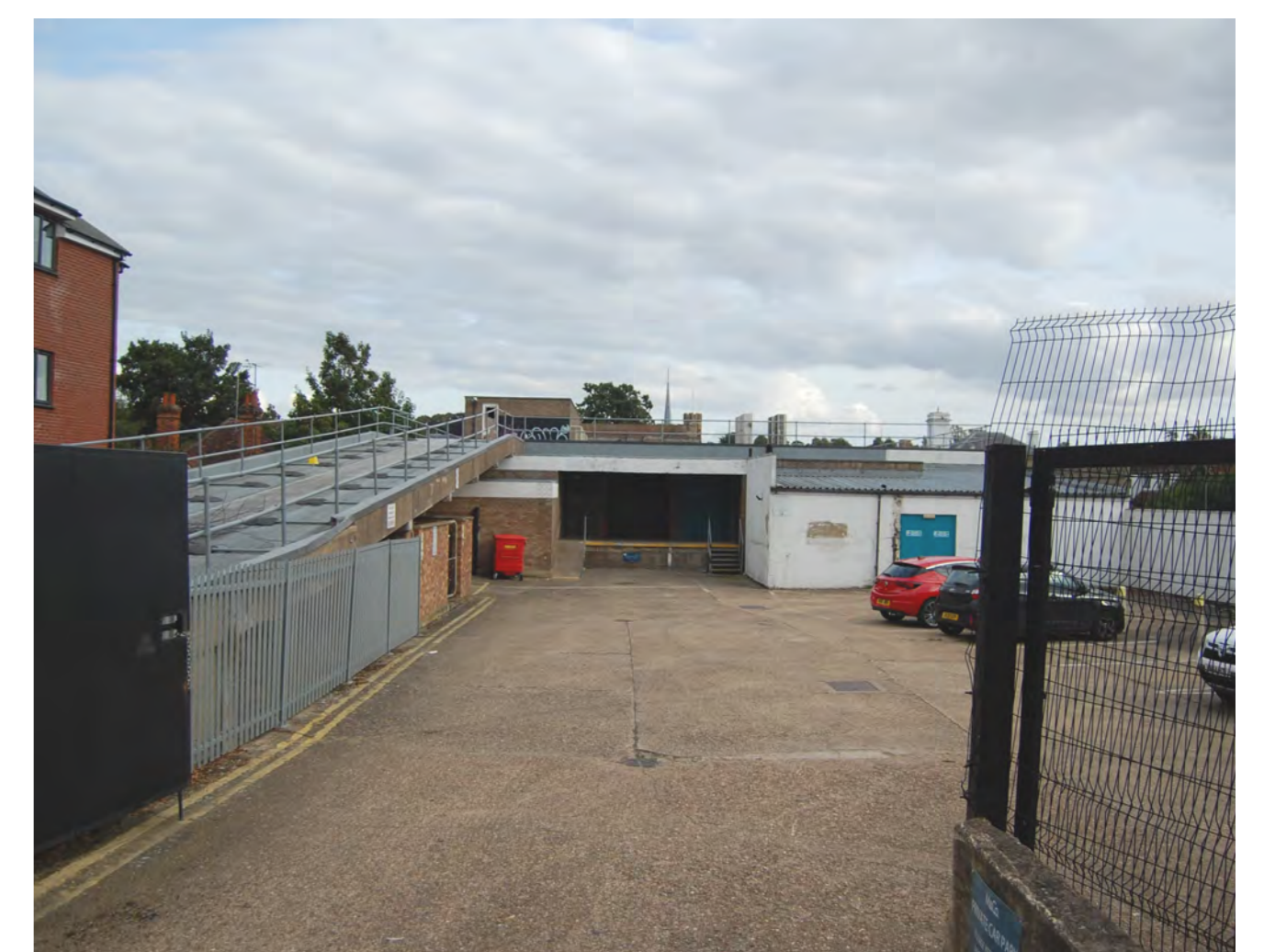
6. Existing Ramp and Carpark
